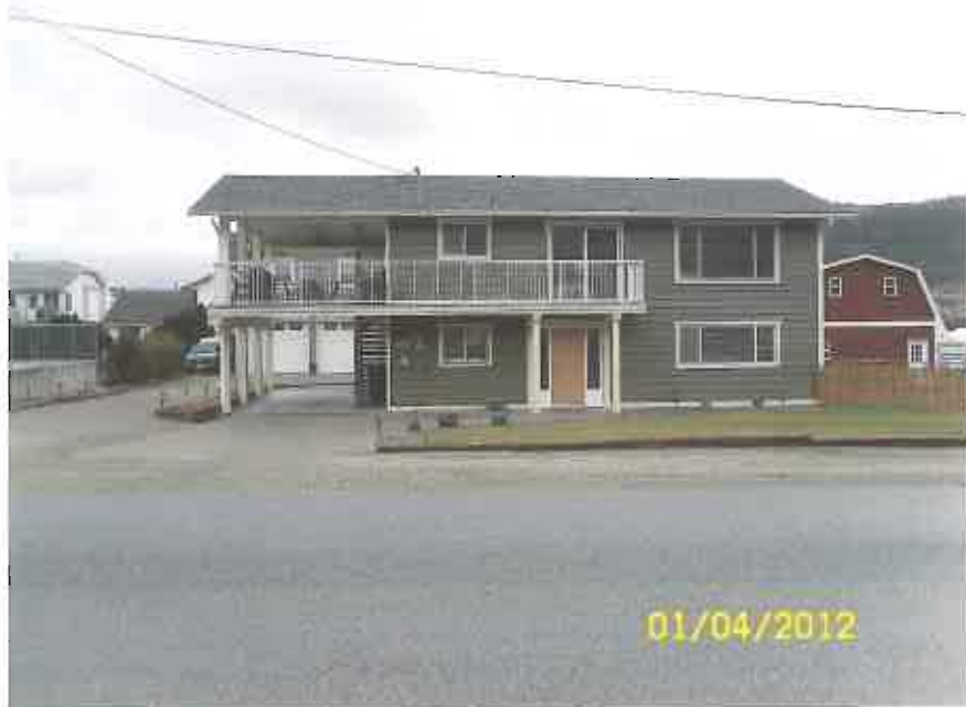
Front of House (facing Yates)
