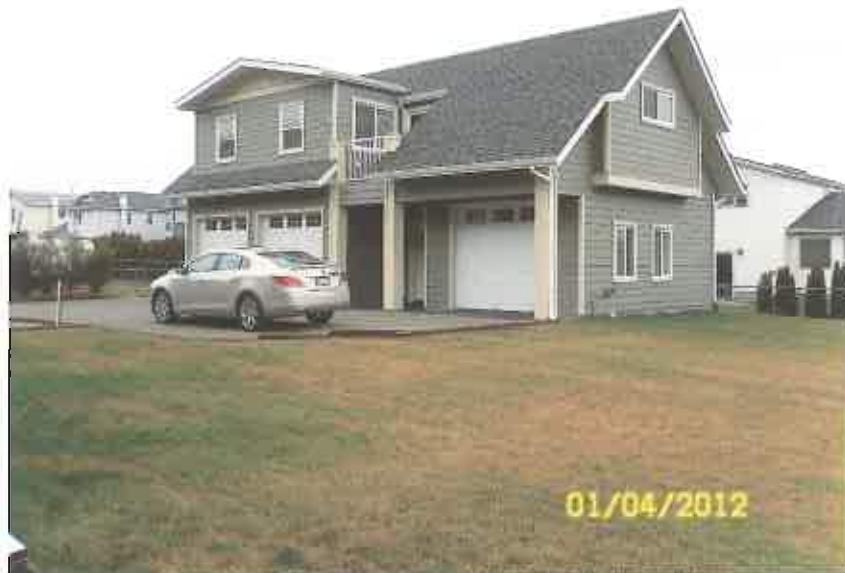
Front of Garage (facing rear of existing house)
